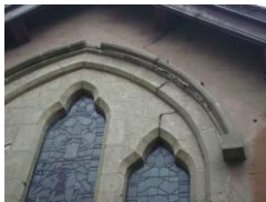
Movement cracks
